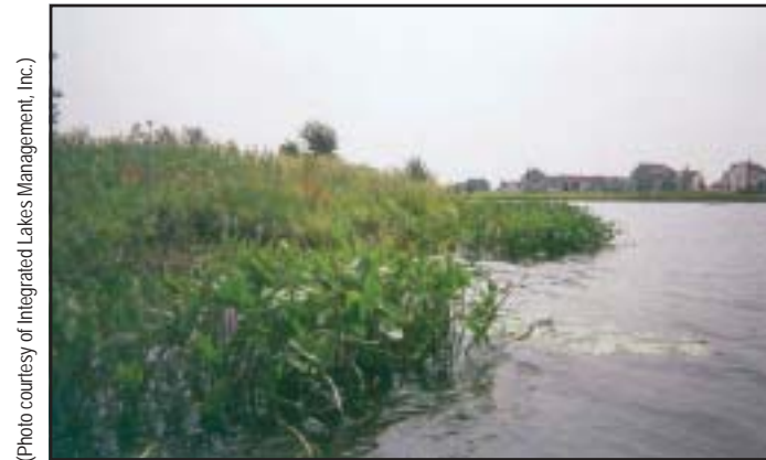
Native vegetation was used on this wet basin bank stabilization project in Lake County.
